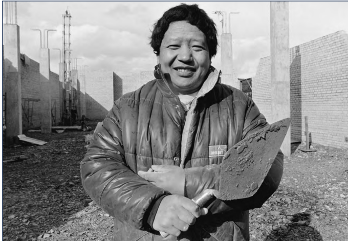
Akong Rinpoche on the Samye Ling Temple building site
